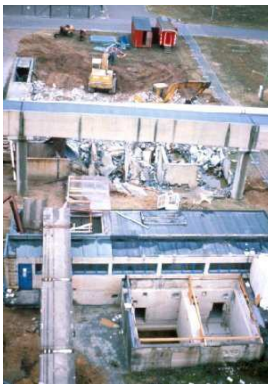
Figure 1. Demolition of buildings 6A/6B
