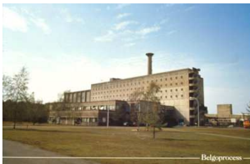
Figure 3. Main process building of the former Eurochemic reprocessing plant
