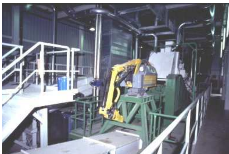
Figure 4. General view of the concrete crushing and sampling facility
