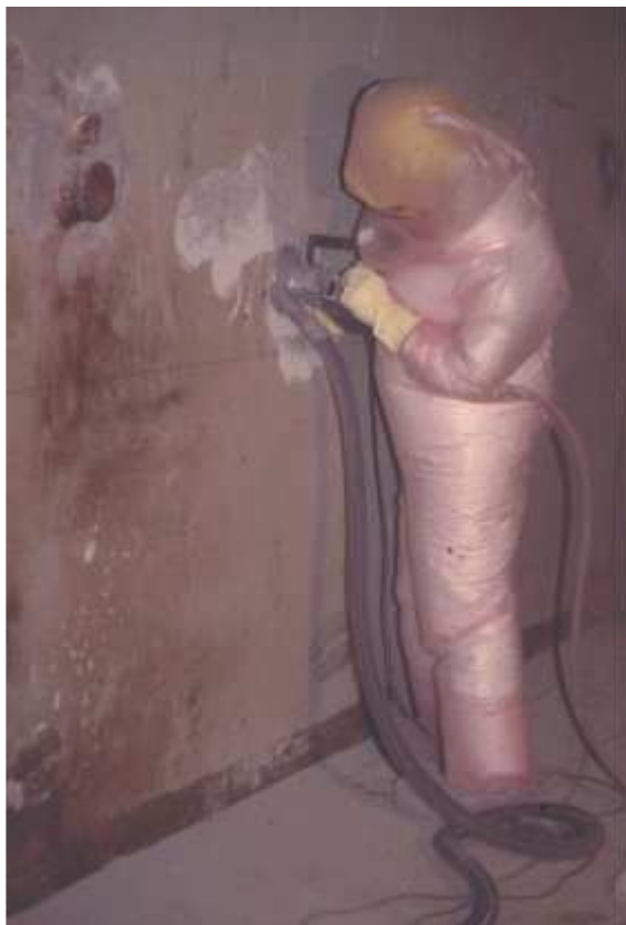
Figure 2. Handshaver for concrete decontamination
