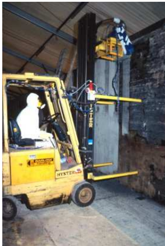
Figure 3. Milling cutter for concrete decontamination
