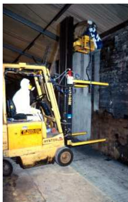
Figure 4. Removal of bitumen layer
