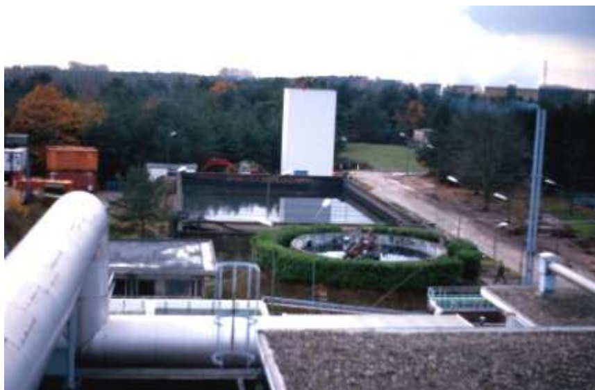
Figure 1. Open storage pond in original status
