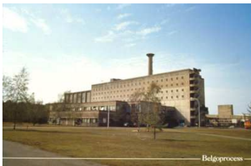
Figure 1. Main process building of the former Eurochemic reprocessing plant
