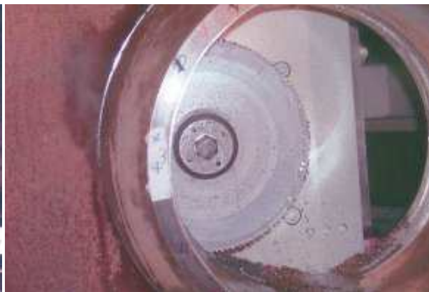
Figure 14. Cutting of a reactor coolant pipe nozzle
