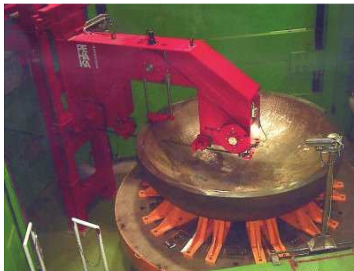
Figure 10. Segments cut into RPV bottom with band saw
