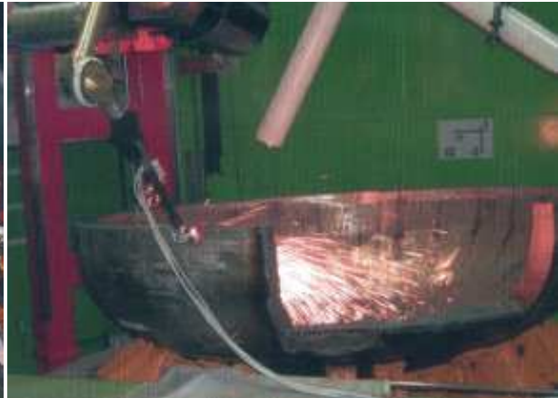
Figure 12. Cutting of vessel bottom with oxyacetylene burner
