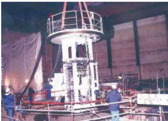
Figure 13. Moving of the milling facility into RPV 7
