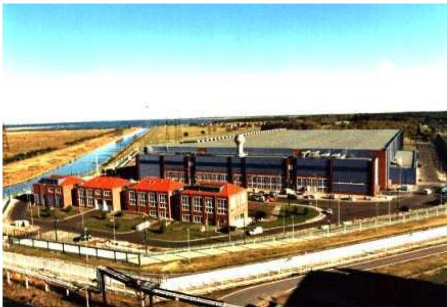
Figure 2. Sight view of the Interim Storage North (ISN)
