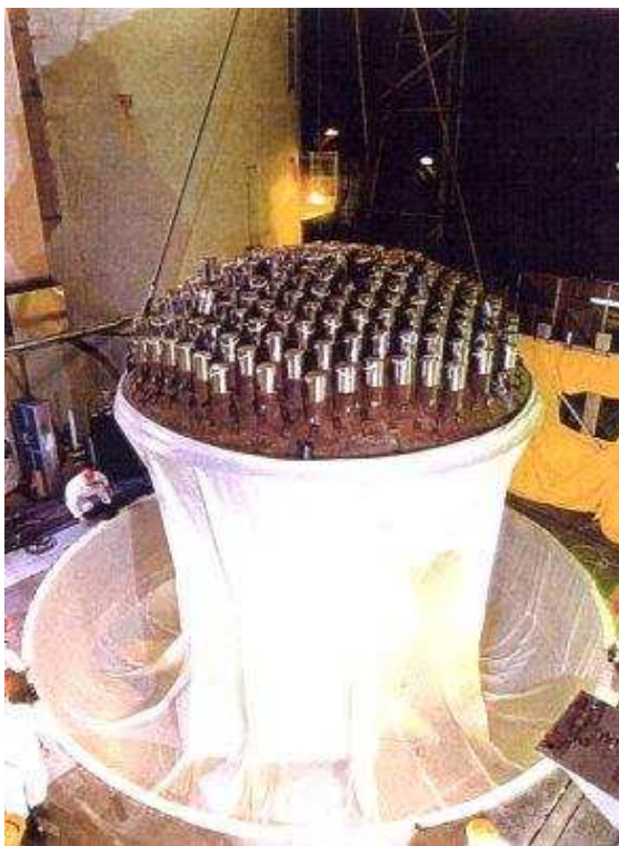
Figure 9. Flexible membrane attached around the cut section
