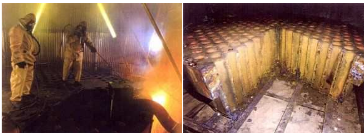
Figure 4 and 5. Dismantling of the Top Biological Shield
